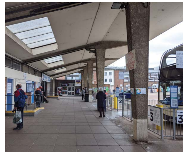
Finish at Exeter bus station.
