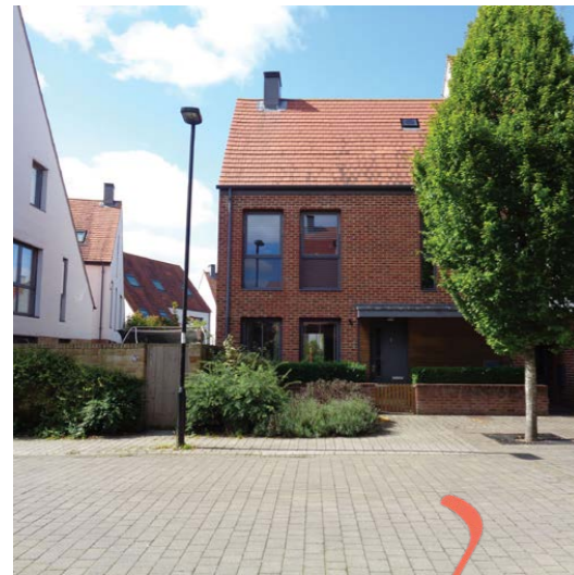
The architecture was varied and included small and larger homes, as well as flats.
